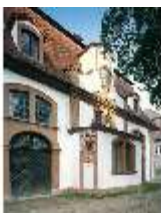
Ell.I, Reithalle, Ostfassade, DE003107, BSV-
